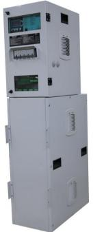
1110XX is the DC Supply system, is used for to supply DC to Scada, measurement, protection and MV Switching Equipments in OG Switching Centers.
